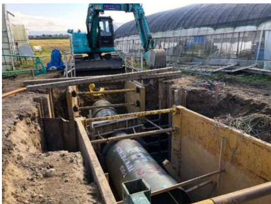
FRPM管布設状況①
