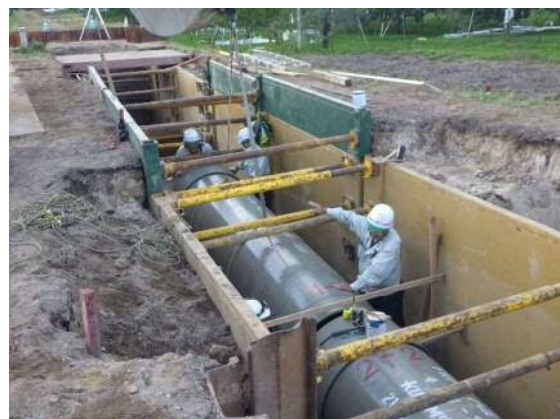
FRPM管布設状況②
